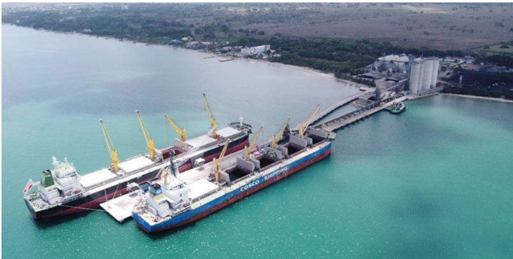
Figure 18.5 – Port of Tolú Facilities
